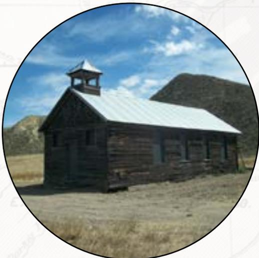
The Collins Schoolhouse in Loma put on a new roof and applied wood preservative to the walls to help prevent further deterioration.
